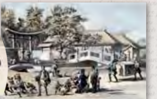
BRIDGE OF CUT STONE & ENTRANCE TO A TEMPLE, SIMODA.
